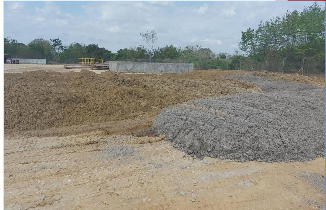
Free water is rapidly transferred to the environment allowing rapid dehydration of the cuttings.
